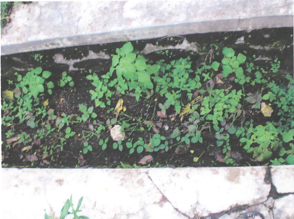
Saluran Drainase Ksatrian Kiri
