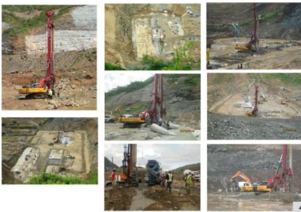
Fig. 6. The Construction of DAM Diaphragm wall
