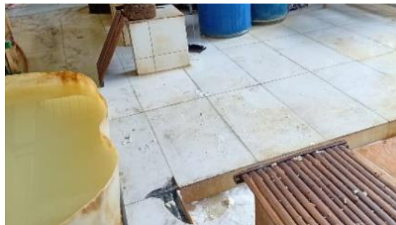
Gambar 1.4 Lantai area kerja
