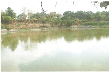
Gambar 28 Check Dam Tanjungan
