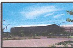
Parkir inner court yard
