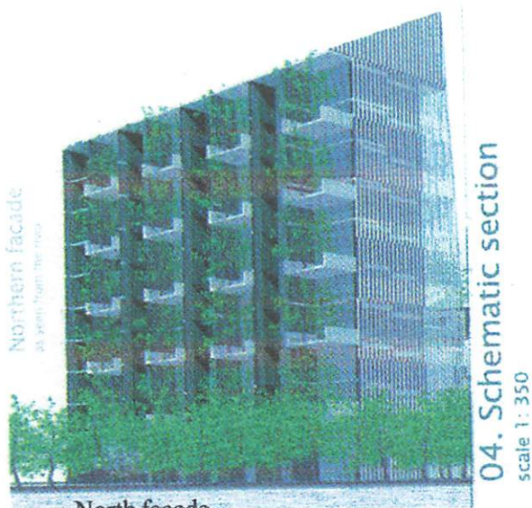
North façade As seen front the river.
