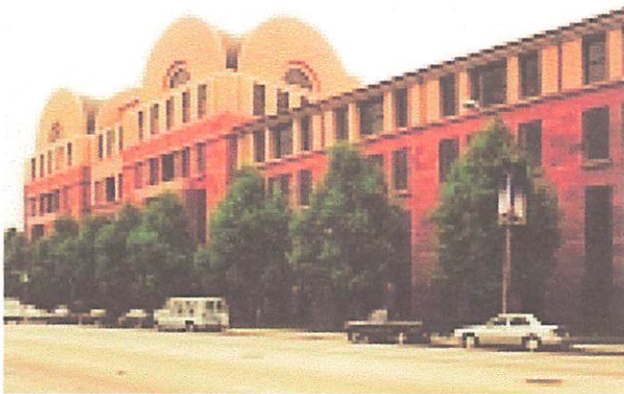
( Gambar 3.8 Tampak samping Team Disney Building)
