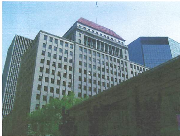
Gbr. 3.3 Portland Public Building Style.
