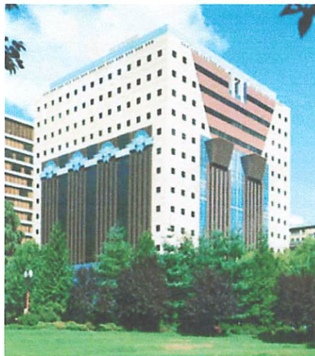
Gbr. 3.2 Portland Public Building, Oregon
