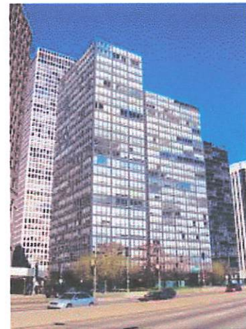
Gambar 4 : Lake Shore Drive apartments Chicago, Illinois (1949 – 1951)
