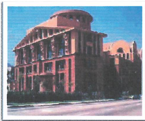
Gambar 2.2. Team Disney Building , Burbank – California
