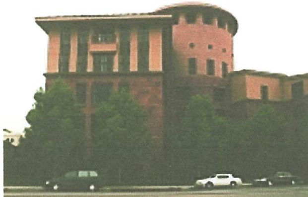
Gambar III.9: Tampak belakang Team Disney Building.
