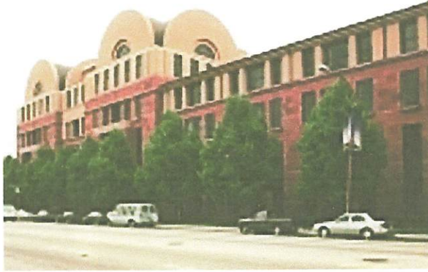
Gambar III.8: Tampak samping Team Disney Building.
