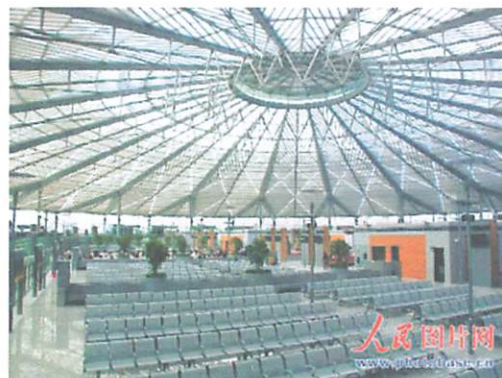
Gambar : Interior Shanghai Sout Stasion, Cina
