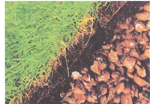
Side of the grass-growing concrete
