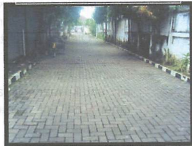
Gambar 4.6 Jalan Paving Block
