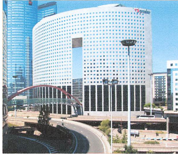
Gambar 2.3 Tampak Depan Pacific Tower
