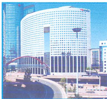
Gambar 20. Fasad Gedung Pacific Tower.
