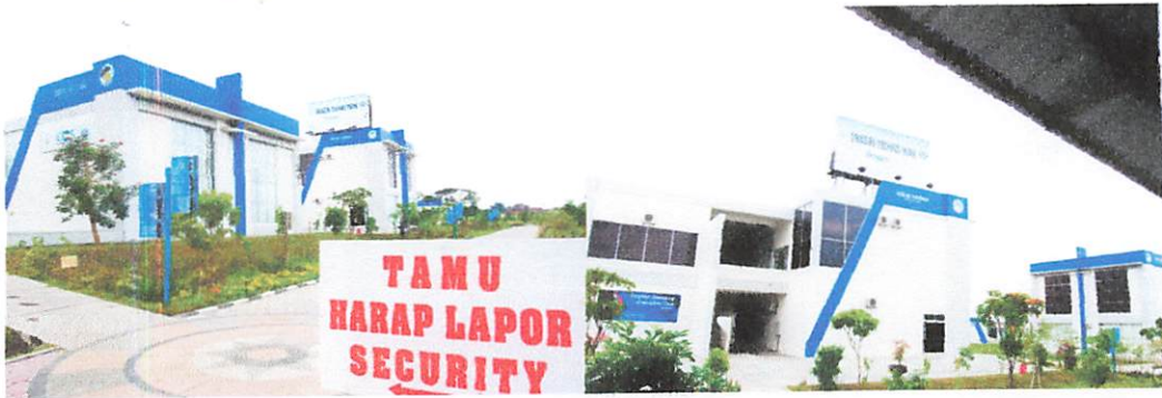
Gambar 2.1. Technopark Sragen Sumber: Survey 2010
