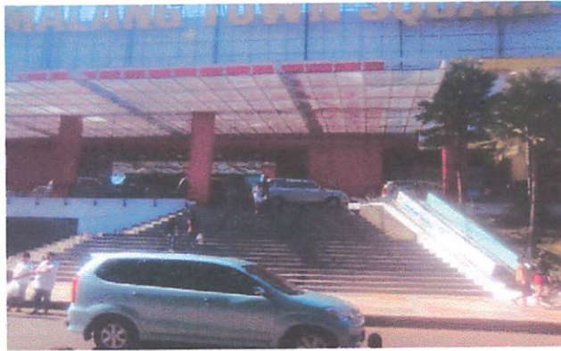
(tampak depan Malang Town Square)
