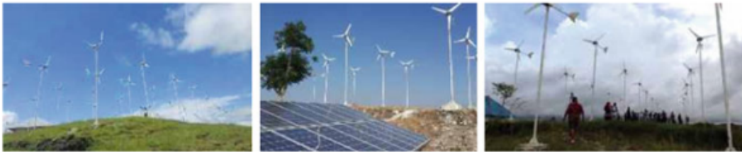
Fig. 19.6 Wind energy farm at Kamanggi
