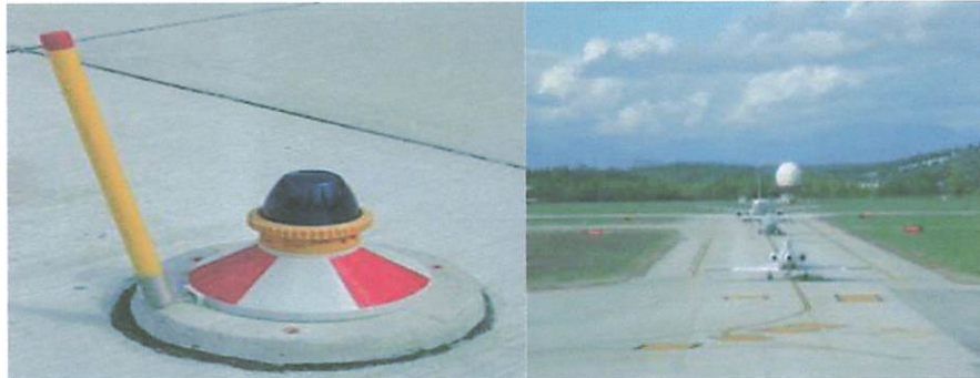
Gambar 2.6: Lampu Lampu Taxiway
