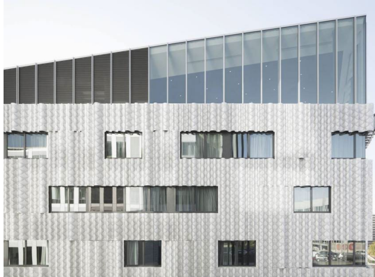
Gambar 2. 34. Detail Kemiringan Hotel Sumber : Archdaily, 2017
