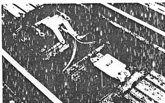
FIGURE 14.—Track Circuit Wiring
