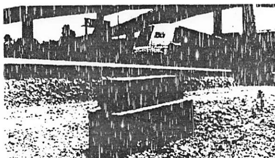
FIGURE 15.—Wayside Equipment Case (contains multiplex equipment for transmitting information between trains and station control rooms)
