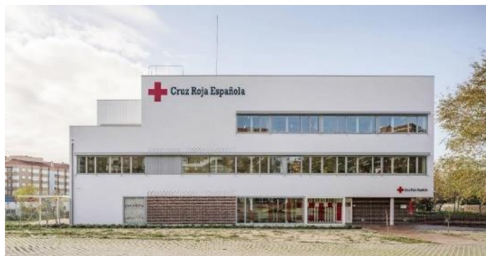
Gambar 2. 19 Tampak Depan Spanish Red Cross Headquarters
