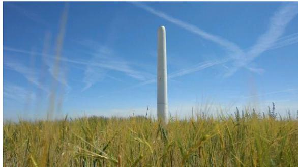
**Gambar 9. Vortex Bladeless Wind Turbines**
