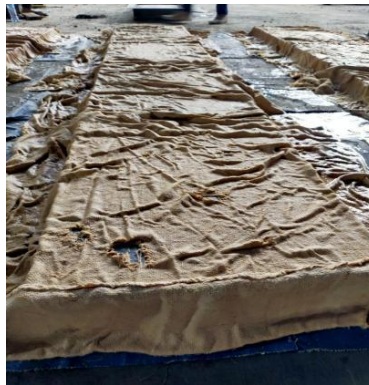
Gambar 3. 8 Proses Perawatan Beton
