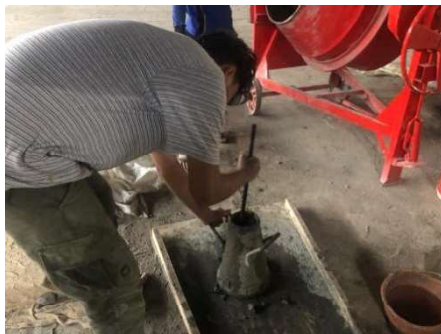
Proses pengujian slump
