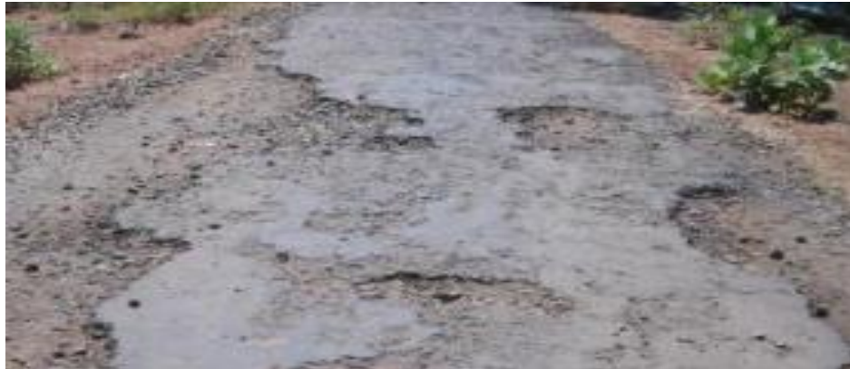
Gambar 2. 11 Disintegrasi ( Disintegration )
