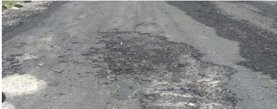
Gambar 2. 13 Agregat Lepas ( Raveling )
