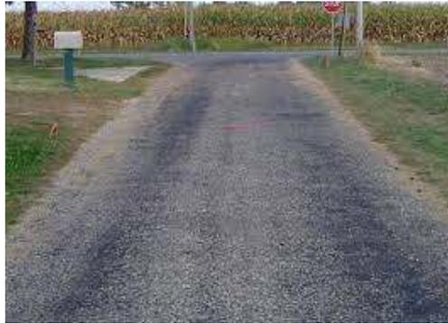
**Gambar 2.10 Pengausan Agregat (Polished Aggregate)**
