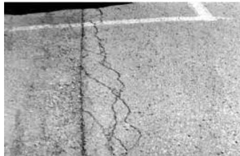
**Gambar 2.8** Retak Sambung (Joint Reflection Cracking)
