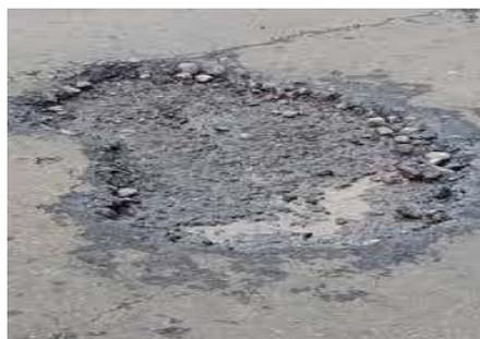
**Gambar 2.11 Lubang (Potholes)**
