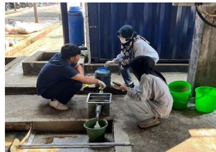
Gambar (4) Running Grease Trap
