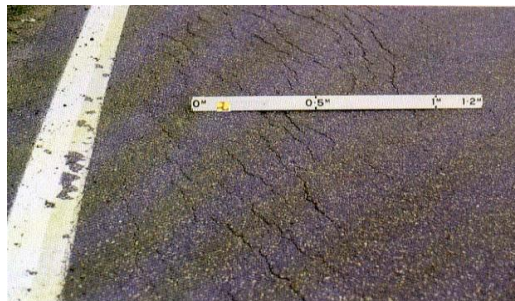
Gambar 2.46 Slippage Cracking
