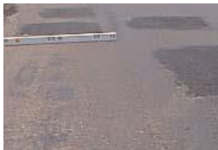
Gambar 2.35 Patching and Utility Cut Patching
