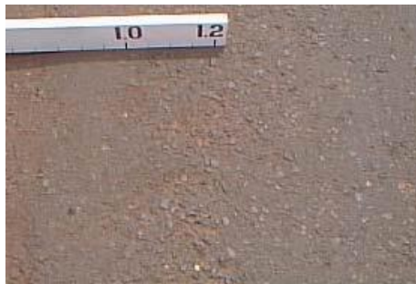
Gambar 2.37 Polished Aggregate
