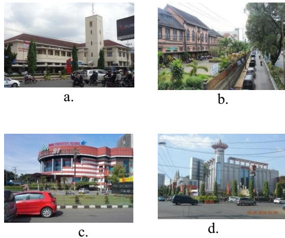
Figure 3. (a). PLN office, (b). Frateran Junior High School, (c). Dieng Plaza, (d). Sarinah. Source: Field Survey, 2013
