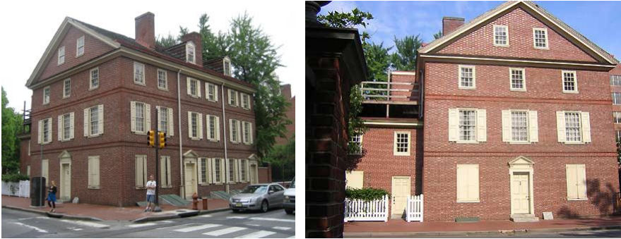
Gambar 3.5 Contoh bangunan bergaya Amsterdam school yaitu Dolley Todd House di Philadelphia
