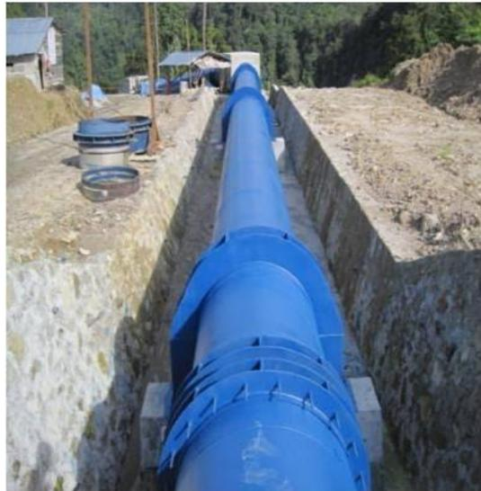
Gambar 2.5 Pipa pesat (penstock)
