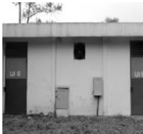
Gambar 2.5 Gardu beton (1)
