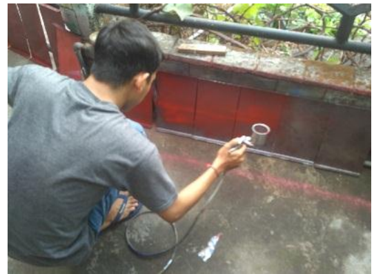
proses pengecatan sudu turbin
