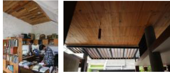
Gambar 7. Penerapan material plafond kayu (Survey Lapangan, 2019)
