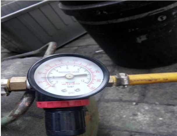
Tekanan proses sandblasting
