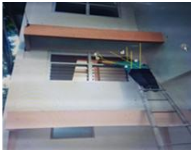
Figure 1b. Cleaning Workers Posture
