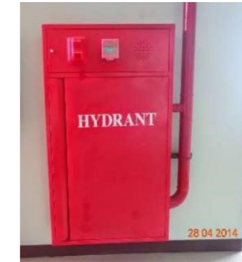
Gambar 4.21 Fire Hydrant Sumber : http://2.bp.blogspot.com/
