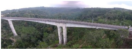
Figure 9 Existing Tukad Bangkung Bridge
