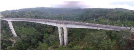
Figure 9 Existing Tukad Bangkung Bridge
