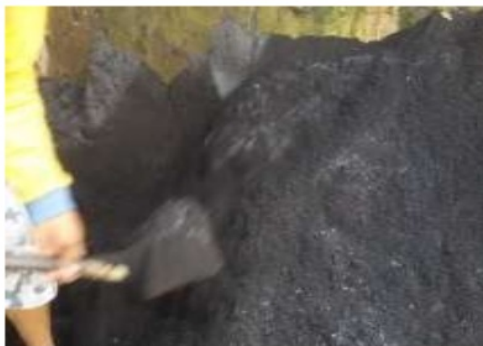
Fig. 4. The collection of concrete sand as filter material
