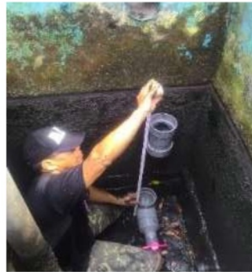
Fig. 15. The installation of filter
