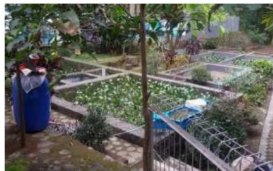
Fig. 1. The condition of communal wastewater plant (IPAL) Tlogomas Malang
