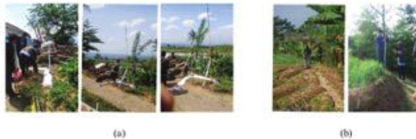
Figure 3: GPS-RTK measurements on control points: (a). GPS base station, (b). GPS rover observing control points.
