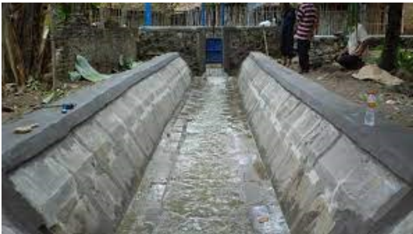
Gambar 2.10 Lining Beton
