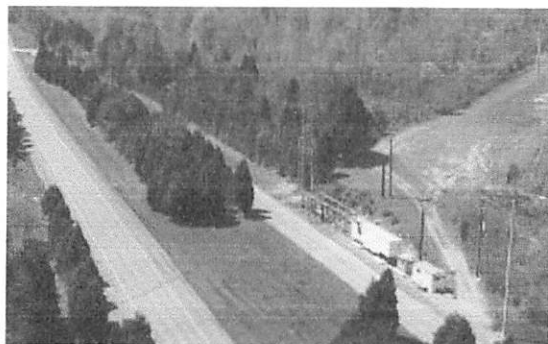
Figure 1. Aerial view of PCAT including its power supply and instrumentation trailers, transmission line structures and current conductor under test.
