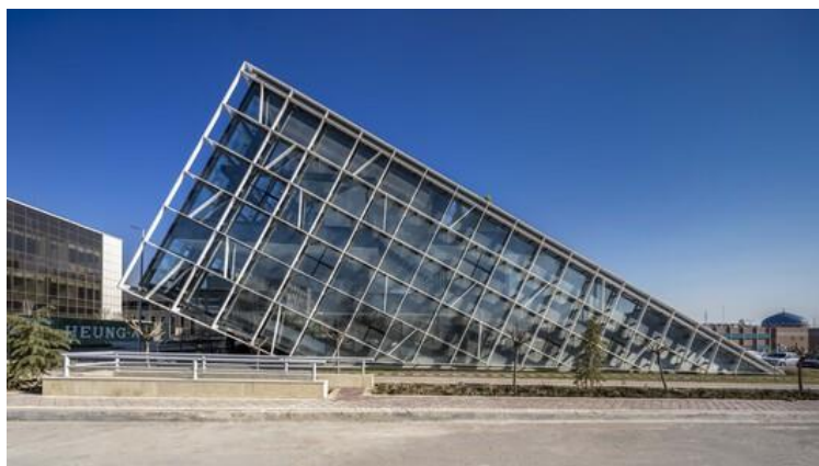
Gambar 2.43 Turbosealtech New Incubator and Office Building, Iran Sumber: (Archdaily, 2022a)
