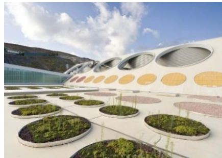
Gambar 2. 24 Atap Waste Treatment Facility
