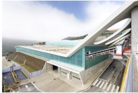
Gambar 2. 22 Waste Treatment Facility
