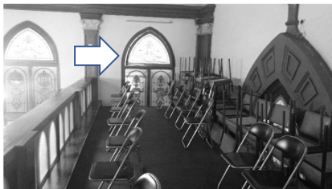
Figure 7. Southwest Balcony Conditioning Location
