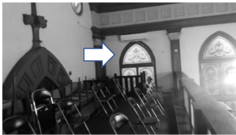
Figure 6. Northwest Balcony Conditioning Location
